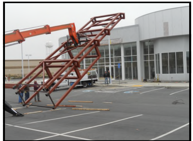
Moving the tower towards the building.
