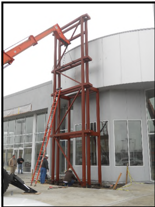
Anchoring the tower to the building. John Gonsalves is off to the left, supervising (of course).
